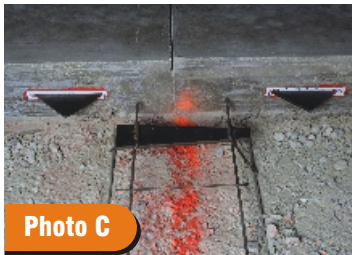
Photo C Tapered plate dowel basket at saw-cut contraction joints and diamond-shaped plate dowels used at the construction joint.
