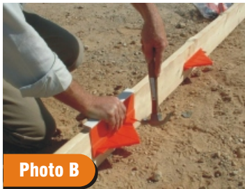
Photo B Installation shot of tapered plate dowels at formed construction joints using installation template.
